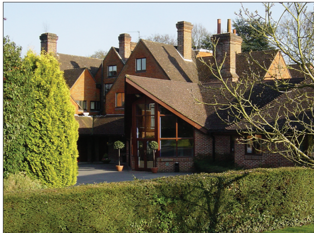
Figure 1: Tadley Court training center
